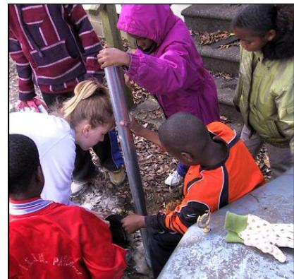
1. Dig a hole for the post. The post needs to be 1.5 to 2 feet underground.
