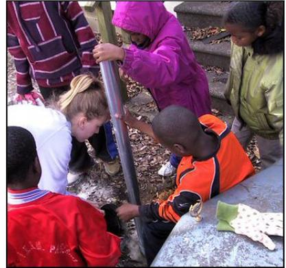
With regular concrete, the post should be set in 24 hours. With quick-set, it will be ready in an hour.
