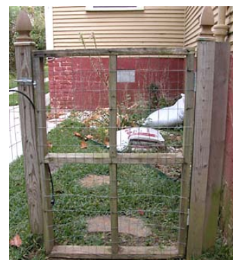
Wood gate with welded wire stapled to it
